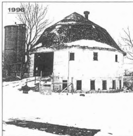
The Dougan barn, anchored by a 14-foot-diameter concrete silo, center, was framed entirely with 2x6s. When it was a working dairy, right, feed drained from the silo to the 42 milking stalls. To move the building, the silo will have to be cut into sections.
