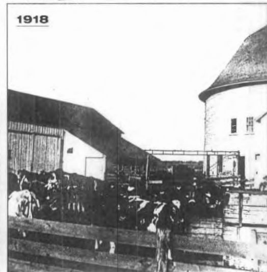
The Dougan barn, anchored by a 14-foot-diameter concrete silo, center, was framed entirely with 2x6s. When it was a working dairy, right, feed drained from the silo to the 42 milking stalls. To move the building, the silo will have to be cut into sections.
